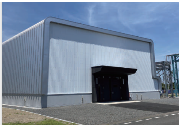
iFactory建屋外観
